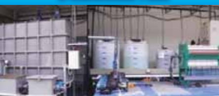
Dissolved Air Flotation Plant
